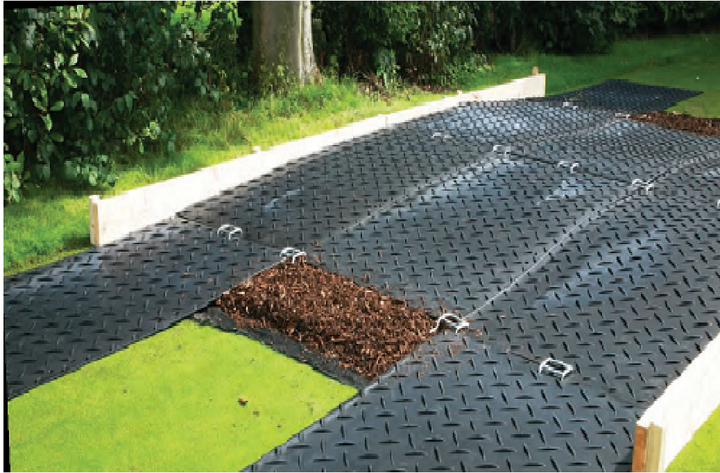
Example of use of steel/road plates over root area.
